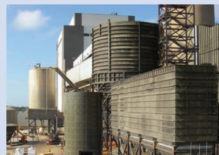
Bolted RTP, Field-weld & Hybrid Tank Construction
