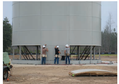
Standpipe - jacked from grade level
