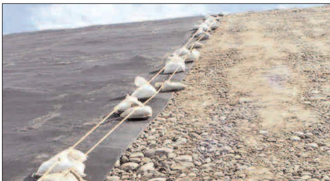
Figure 4 - Use of GSE geotextiles for geomembrane protection.
